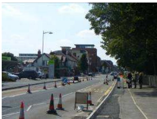
London Road south of the conservation area
