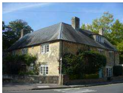
Corallian limestone with a lime render weather coating
