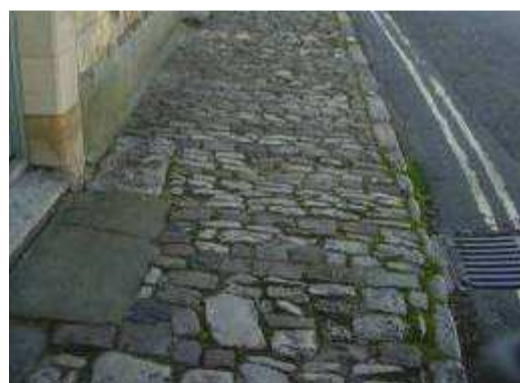
Area of listed Paving at St Andrew's Road
