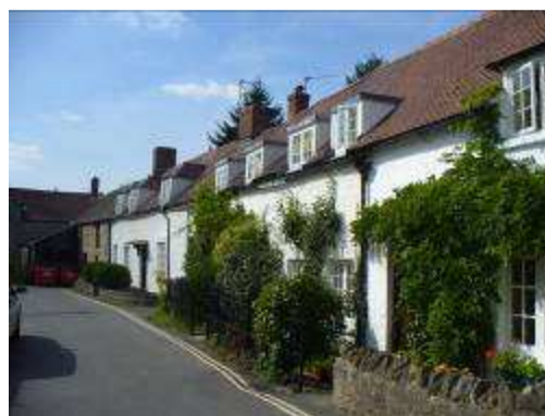
View west along cottage frontage at The Croft
