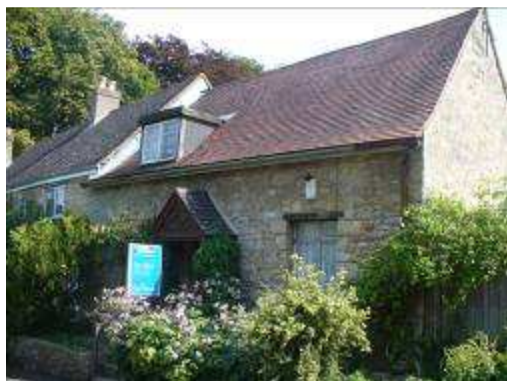
No. 18 St Andrew's Lane a small workers' cottage, probably of 18 th or early 19 th century construction
